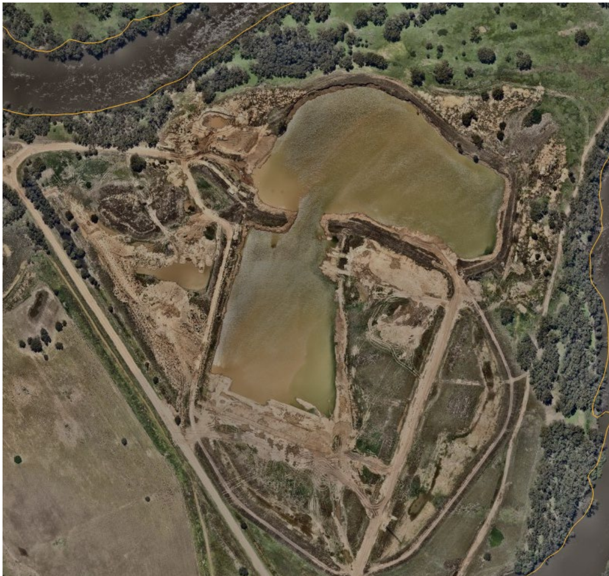
Figure 11: Colapse of wall between Cell 1 and Cell2 – February 2023.
