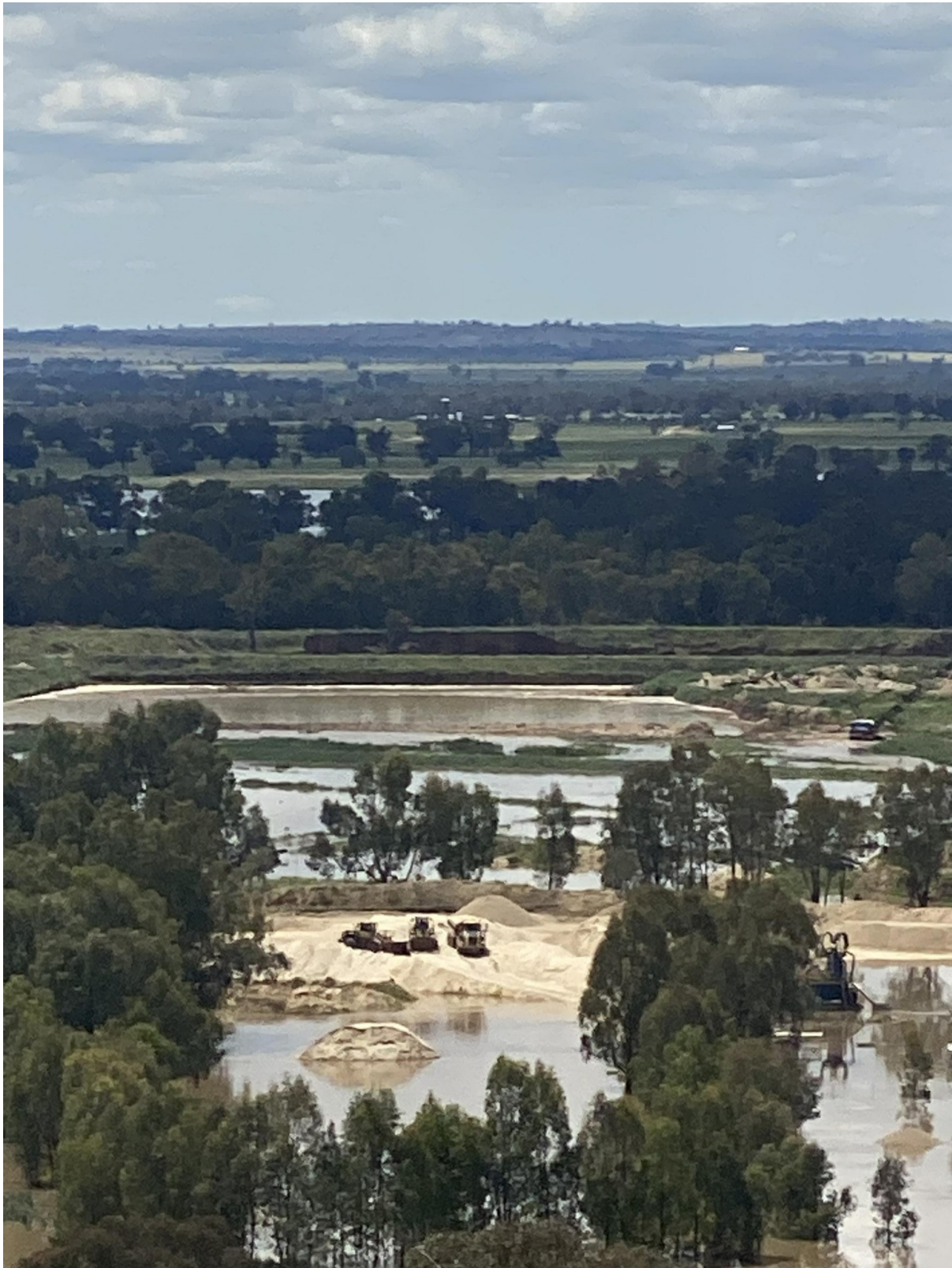
Figure 9: November 2022 Flooding, breach of wall between Cell 1 and Cell 2 (facing North towards active cells and River).
