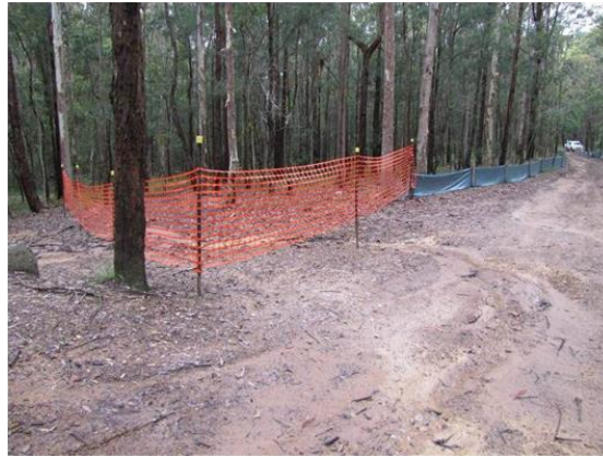
Plate 1 High Visibility Protective Fencing
