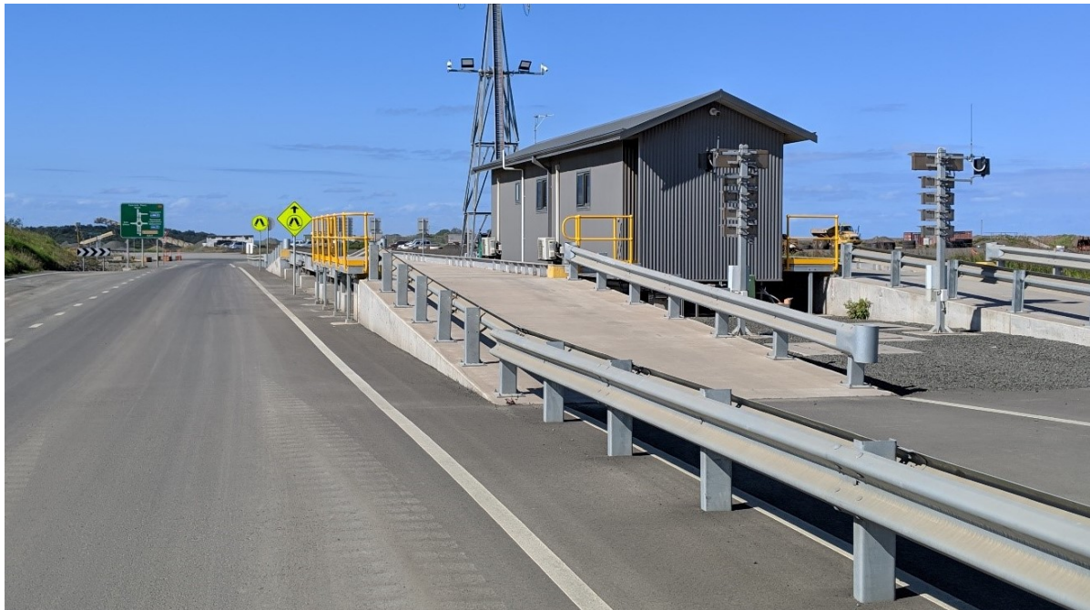
Figure 3: Bass Point Quarry weighbridge (C. Flood, April 2019).
