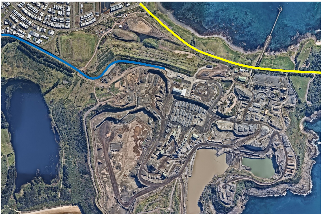
Figure 1: Aerial map of Bass Point Quarry and surrounds (Nearmap, 2021), with the Bass Point Quarry Road site access marked in blue, and the Bass Point Tourist Road site access marked in yellow.
