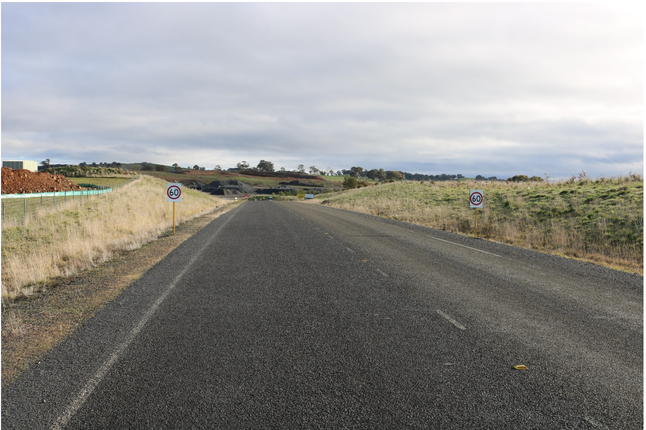
Photograph 1 – Quarry Haul Road
