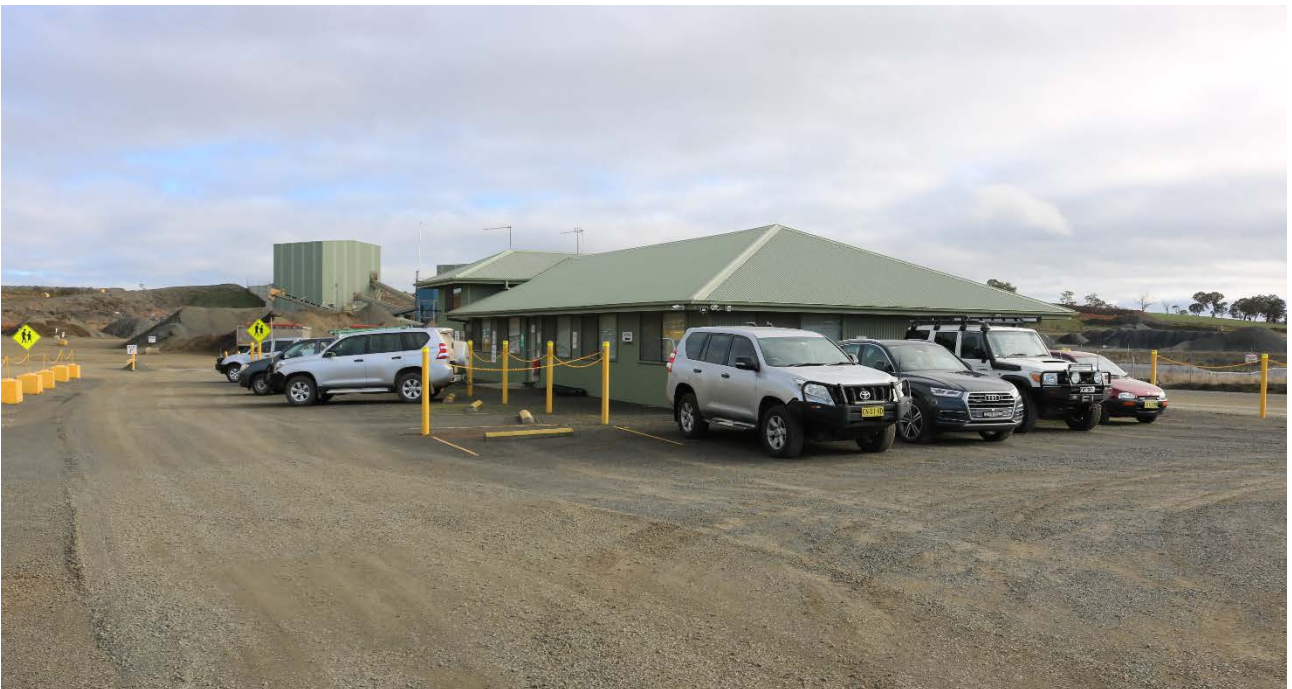
Photograph 3 – Internal Car parking
