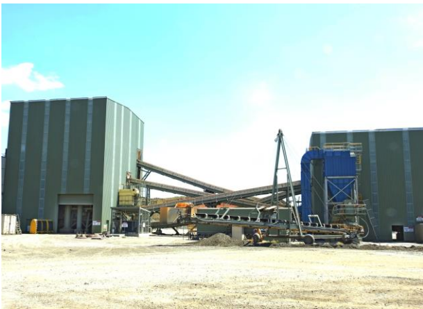
Plate 7: Enclosed primary crusher and secondary screening area – evidence of good practice for dust management (E869K_048)
