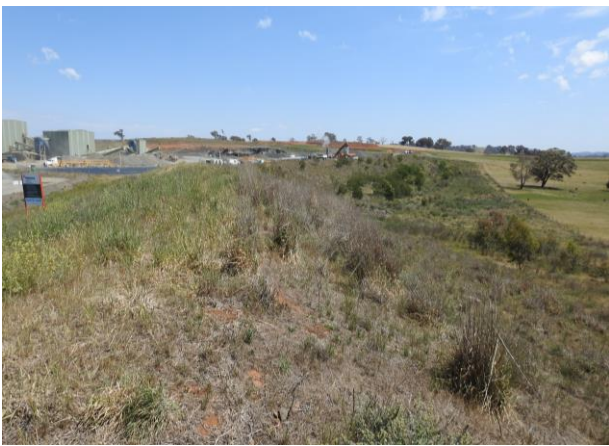
Plate 5: Amenity bunding to the east of the processing and stockpiling area with evidence of successful revegetation (E869K_025)
