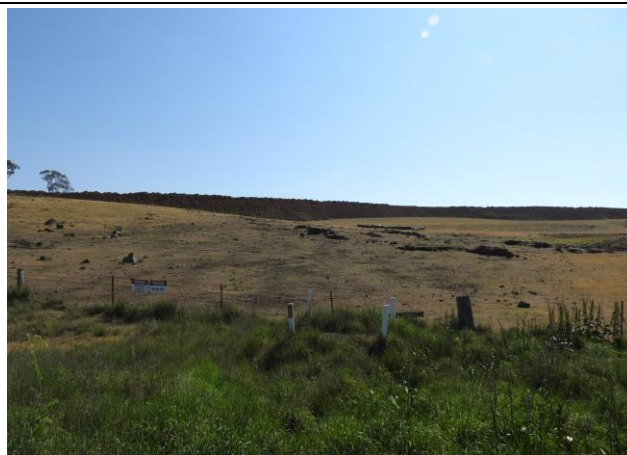
Plate 4: Amenity bunding observed from the Mitchell Highway – no stabilising vegetation (E869K_002)
