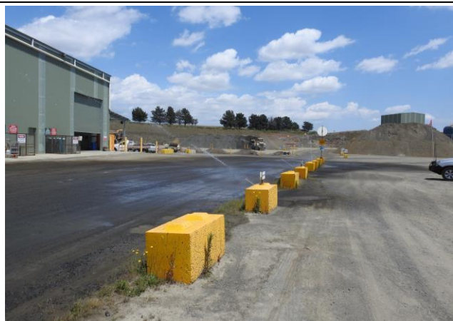
Plate 8: Automatic sprinkling system between administration and weighbridge building and workshop - evidence of good practice for dust management (E869K_062)
