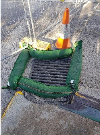
Sediment protection along gutters and around stormwater grates
