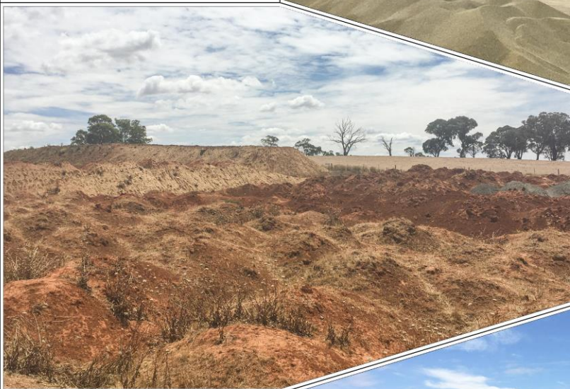
Plate 11: View to the south of topsoil in Growth Medium Storage Area (Ref: Plate 11)
