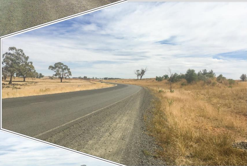
Plate 2: View of amenity bund and tubestock planting along Site Access Road (Ref: Plate 2)
