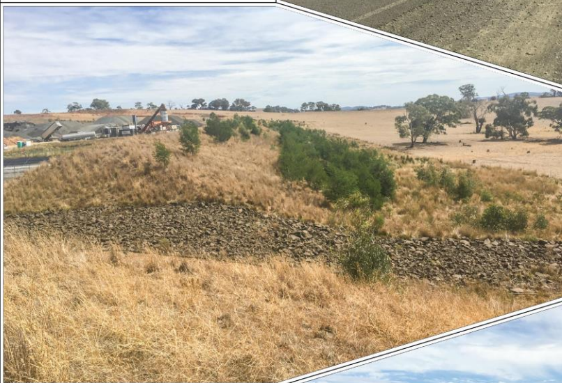
Plate 3: View of tubestock planted on amenity bund along eastern boundary of the Infrastructure Area (Ref: Plate 3)
