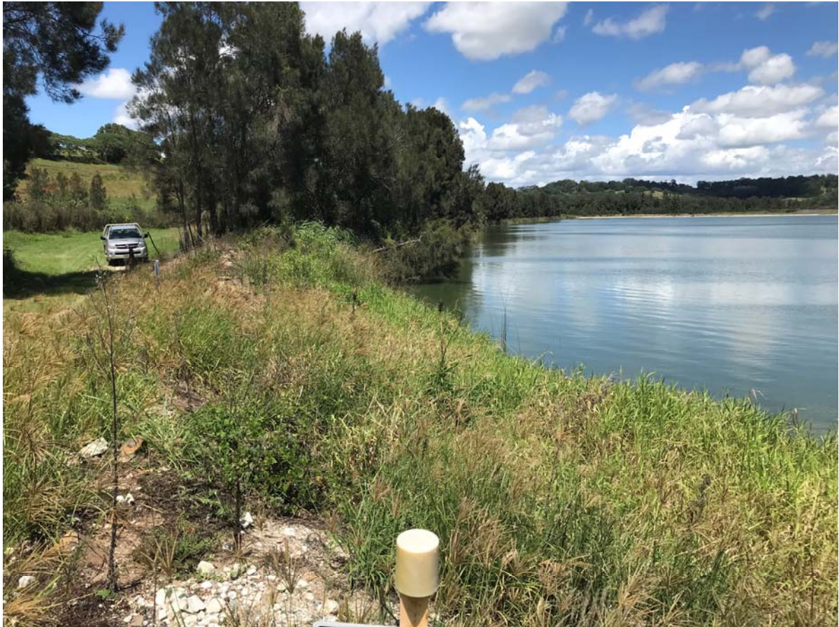
Photo 3.1 - Rehabilitation Area 1 (facing south) February 2018
