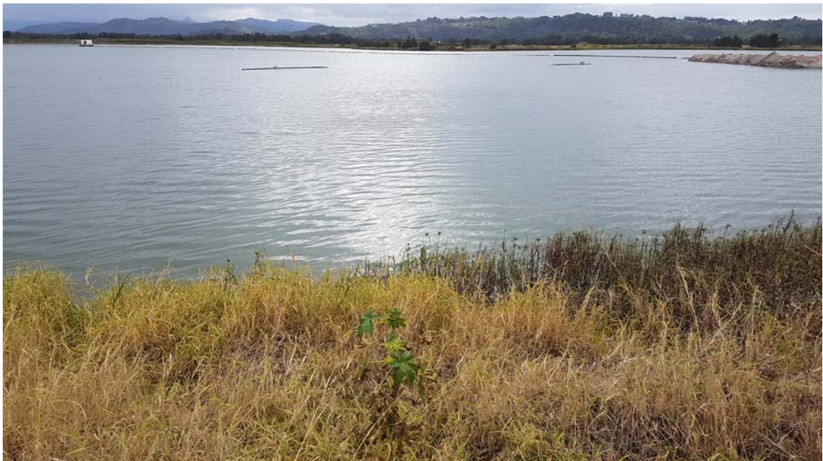
Photo 4.2 - Rehabilitation Area 1 (facing west) September 2018
