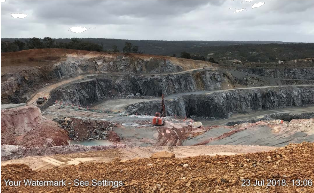
Plate A West quarry pit extension area A, SW elevation
