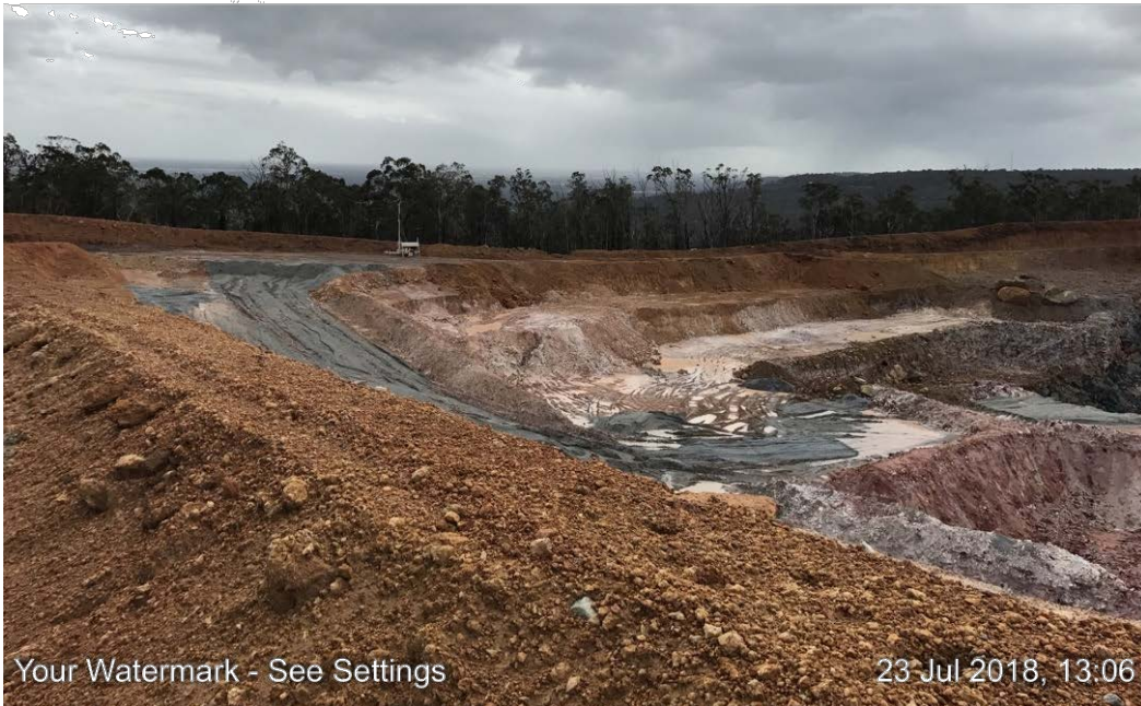
Plate B West quarry pit extension area A, SE elevation
