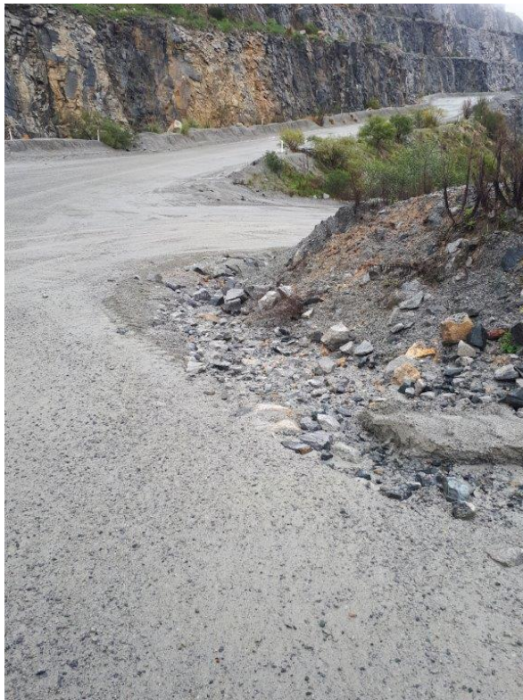
Plate J Drainage channel along secondary road
