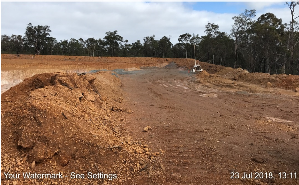
Plate D West quarry pit extension area A, NE elevation
