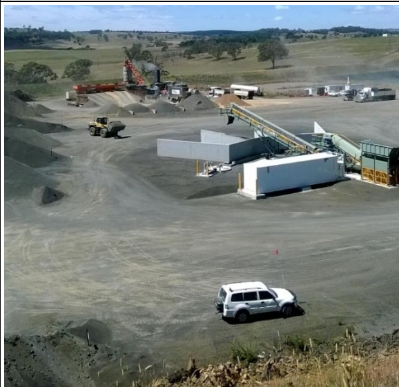
Plate 7 View of the northern section of the Infrastructure Area including the Pre-Coat Plant, various aggregate stockpiles and Pugmill (background) (Ref: E869F_005)
