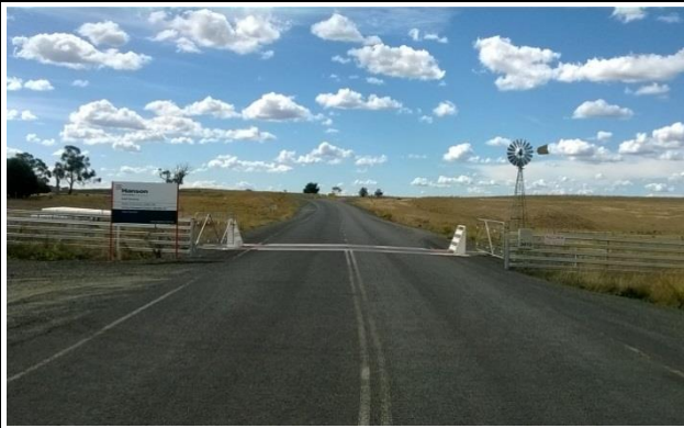
Plate 1 View of site entrance including lockable gate and sealed Site Access Road (Ref: E869G_001)
