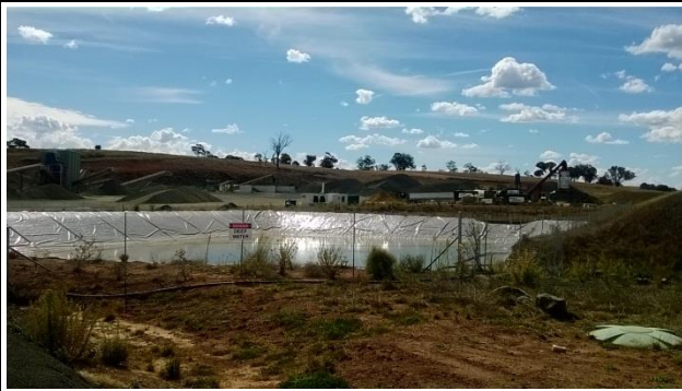
Plate 5 View of Water Storage Dam and Sediment Basin (foreground) with the northern section of the Infrastructure Area in the background (Ref: E869G_004)
