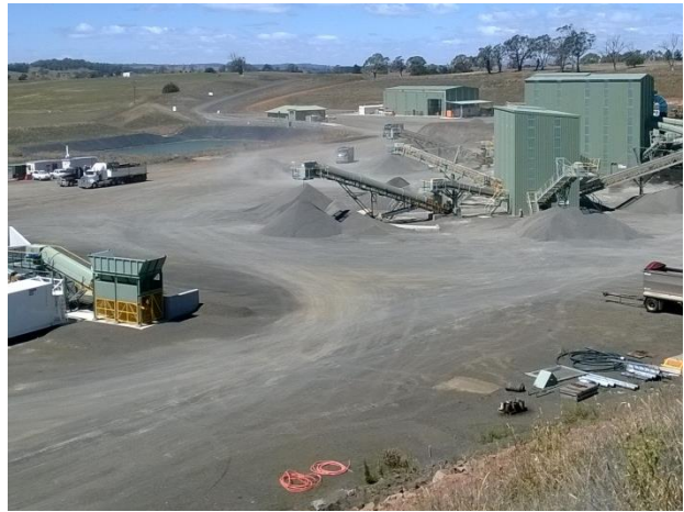
Plate 6 View of the southern section of the Infrastructure Area including the Pre-Coat Plant (left) and Fixed Processing Plant (right) in foreground and Water Storage Dam, Workshop, Site Office and Weighbridge in the background (Ref: E869F_006)
