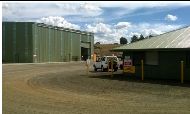
Plate 3 View of Site Office and Workshop buildings (Ref: E869G_003)
