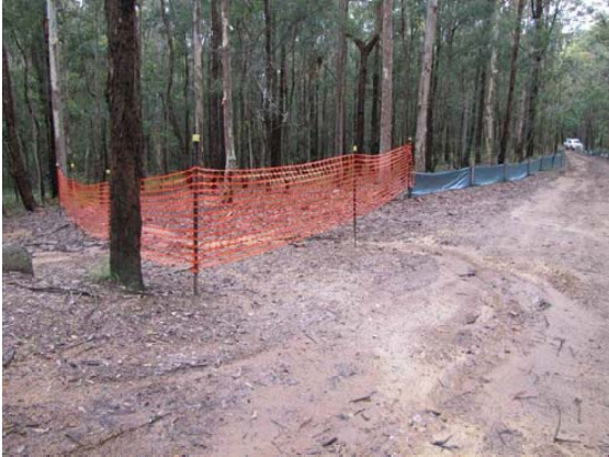
Plate 1 High Visibility Protective Fencing
