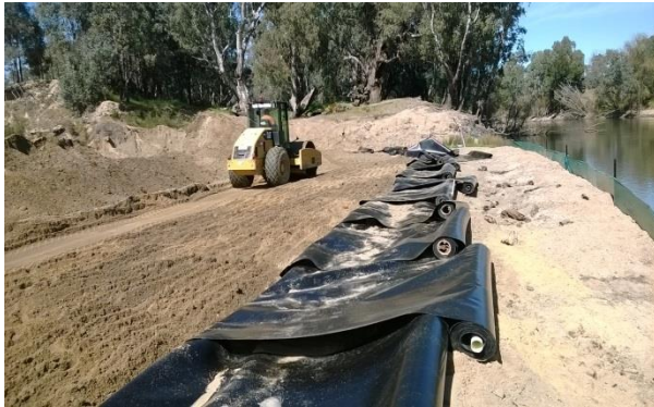
Plate 4.4.5: River bank repair works underway with compacted fill and HDPE liner being installed.
