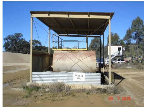
Plate 4.6.1b: Waste oil aboveground tank
