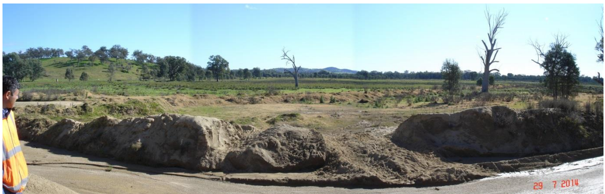
29 July 2014: looking northwest from the process plant and stockpile area to the wetland south of Pit 1. Wash-water from the process plant is directed along a surface channel to Pit 2 for settling and reuse.
