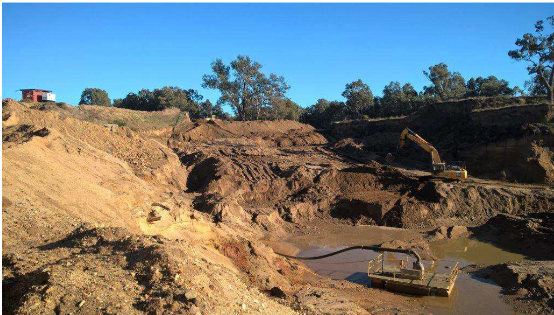
Figure 10: Flood damage repair work to Cell 1 levee
