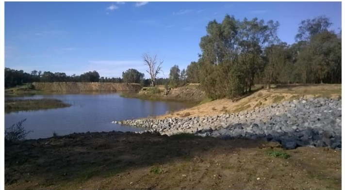
Plate 2: Repaired river bank
